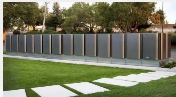
SOFC天然气高温分布式发电
